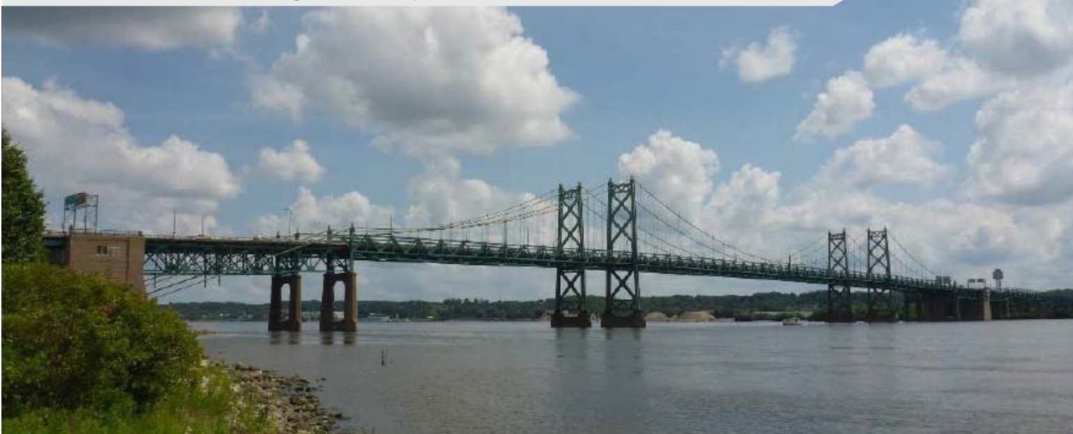
Photo 1: Interstate 74 Bridge in Davenport, Iowa
