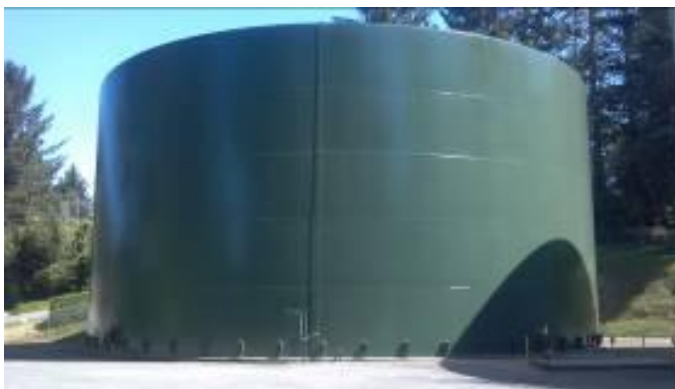
Figure 5. McKinleyville Community Services District 1.5 million gallon water storage tank that was recoated in 2012
