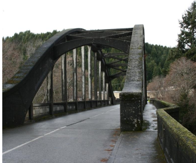
Figure 2. Bridge over North Fork Mad River near Korbel, CA
